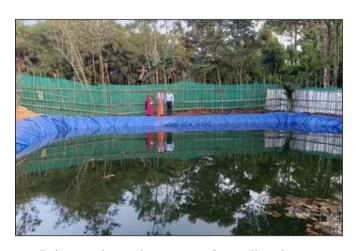
Rain water harvesting structure for small cardamom
